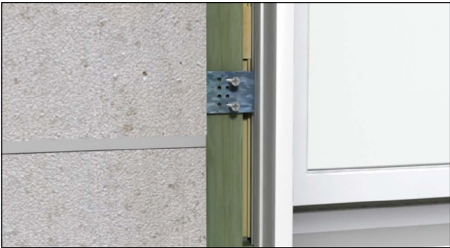
Figure 19 Attaching window with structural brackets.
